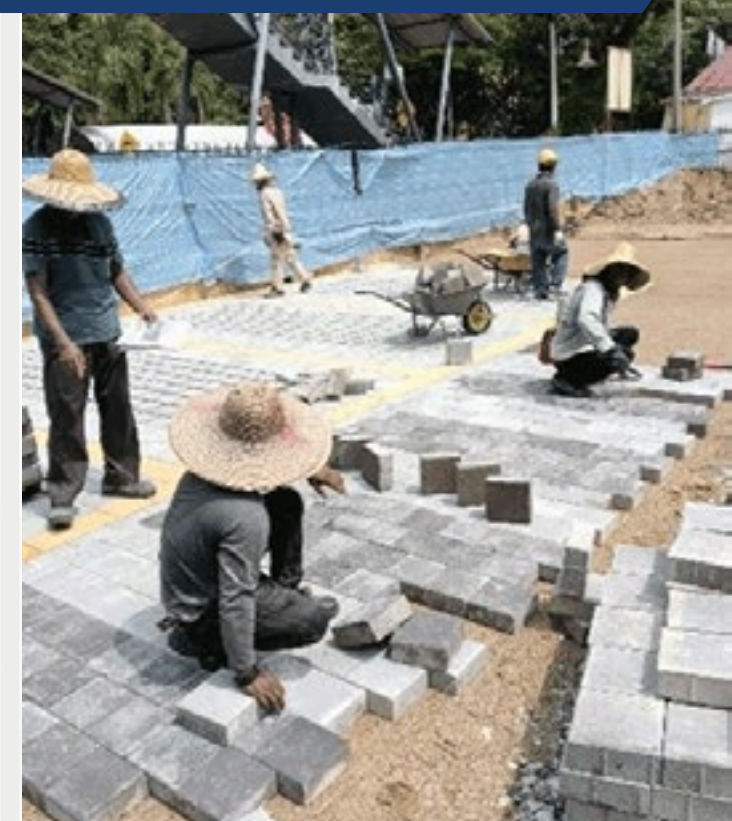
Pavers installation at the car park
